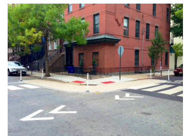
Quick Build Curb Extensions, Princeton, NJ, Credit: WalkBikeNJ.com
