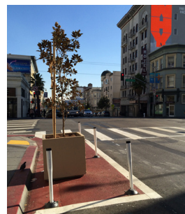
Quick Build Curb Extensions, Princeton, NJ, Credit: WalkBikeNJ.com
