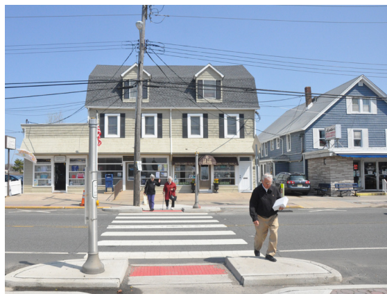
Mid-Block Crossing with curb extensions and signal actuation in Bayhead, NJ
