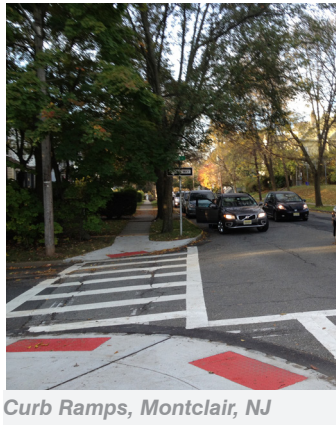
High-Visibility Ladder Crosswalk, Montclair, NJ
